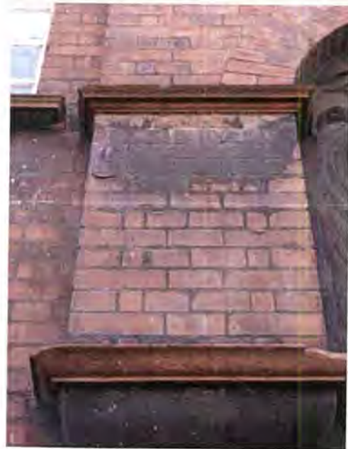
Brickwork stained with heavy sulphur dioxide deposits
