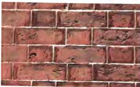
Façade with historic wiggled brickwork
