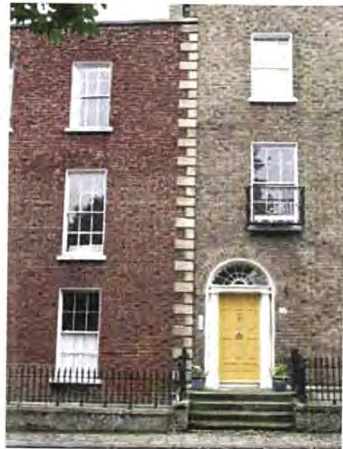
Colour-washed façade brickwork can be seen to the building on the left
