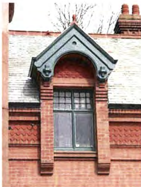
The Red Stables, St Anne's Park, Raheny, Dublin, built in 1886 of machine-made brick from the Portmarnock Brickworks
