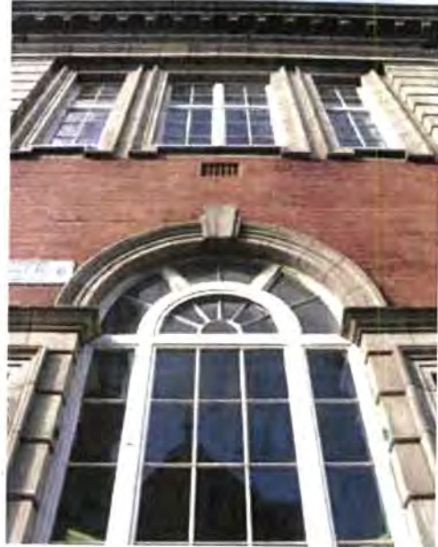
Rathmines Library, Dublin, opened 1913, constructed of Arklow brick and terracotta designed to resemble stonework
