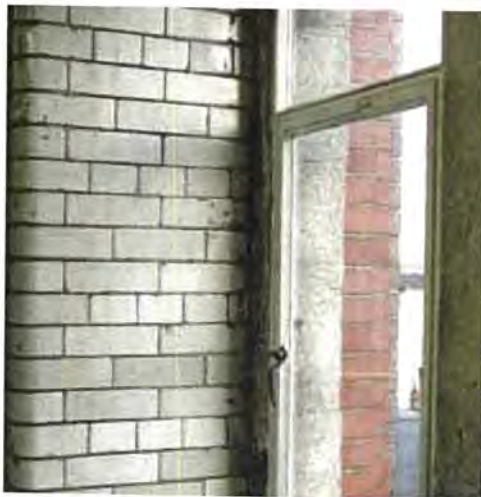
Glazed bricks, in white or pale colours, were often used to the sides of windows and in light wells to reflect more light into the interior of a building
