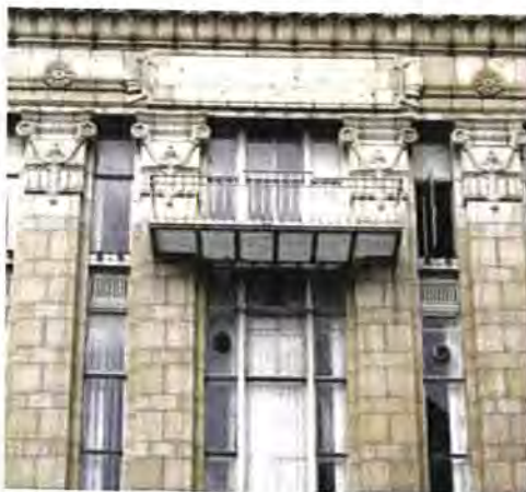
Burton's, Dame St, Dublin, designed in 1929 by Harry Wilson, is an example of high quality faience cladding used to form a giant classical order to the façade
