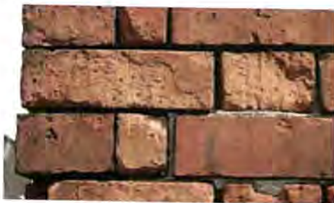
The mortar has weathered back or been washed out of this brickwork to a severe extent and it is now in urgent need of repair and repointing
