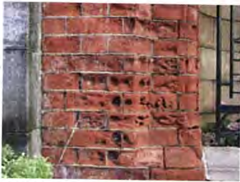
Weathering of brickwork can in some cases be severe. In this case, the decay may have been exacerbated by the mortar being too strong
