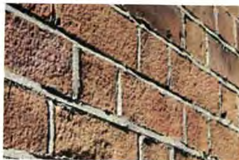
This brickwork shows evidence of damage by over-heavy abrasive cleaning which has removed the fireskin from the bricks making them vulnerable to accelerated decay exacerbated by the cementitious pointing
