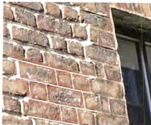
iii) the finished wigging sample
