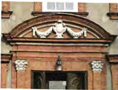
Gauged brickwork of high quality was used in the brick architectural detailing of Beaulieu House, Co. Louth
