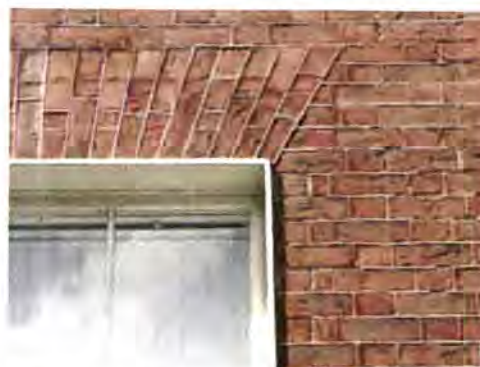
A typical Irish eighteenth-century flat arch window head. It differs from similar English flat arches of the period in that the arch does not splay widely at either end
