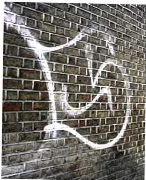
Graffiti on historic brickwork should be cleaned off as soon as possible as it will become more difficult to remove if the paint is allowed to dry and harden. A suitable poultice may be the solution
