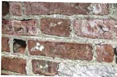
Colour washed bricks with traces of pencilling to the joints at the Hell Fire Club, Desmond's Castle, Askeaton, Co. Limerick
