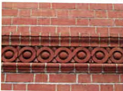
An example of the decorative use of moulded brickwork and terracotta in a stringcourse
