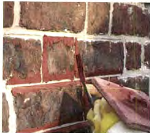
ii) laying in the pigmented stopping mortar up to the ribbon
